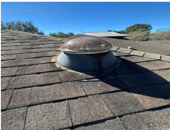
Example of skylight penetration
