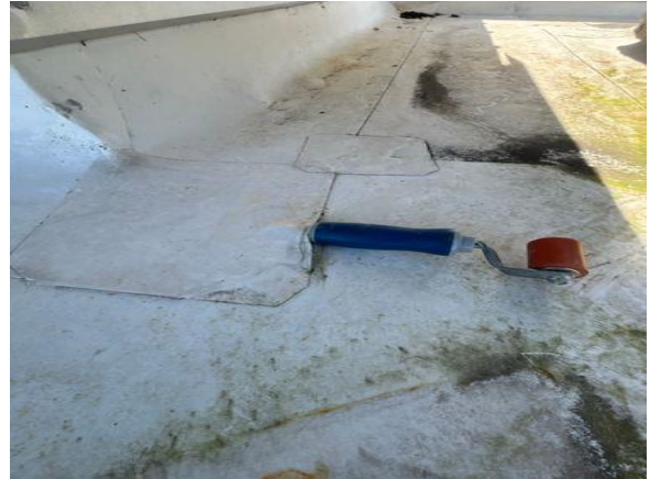
Loose flashing
