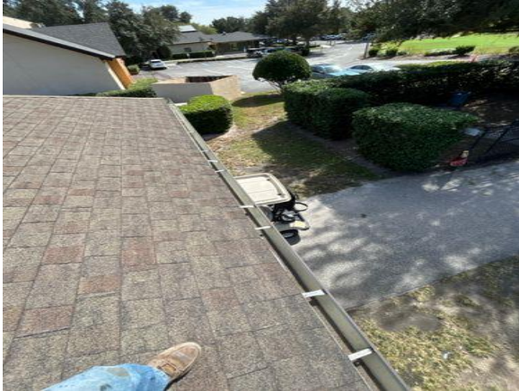
Misplaced gutter brackets
