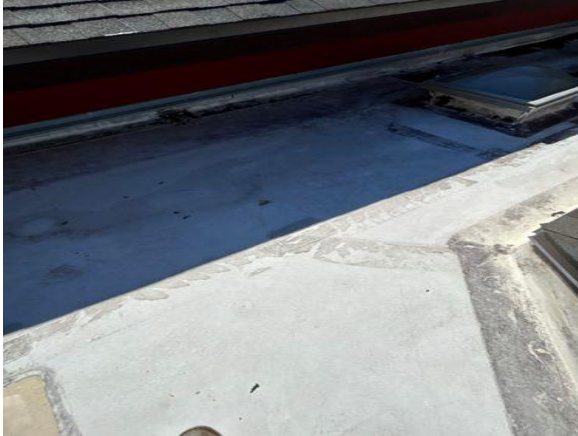
Example of TPO general field and seams
