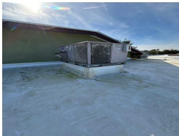
Example of unit penetration
