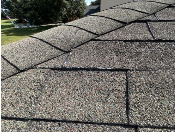
Worn down shingles
