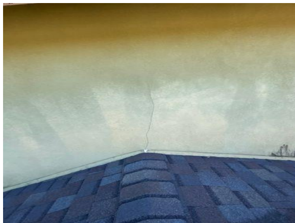
Cracking on siding
