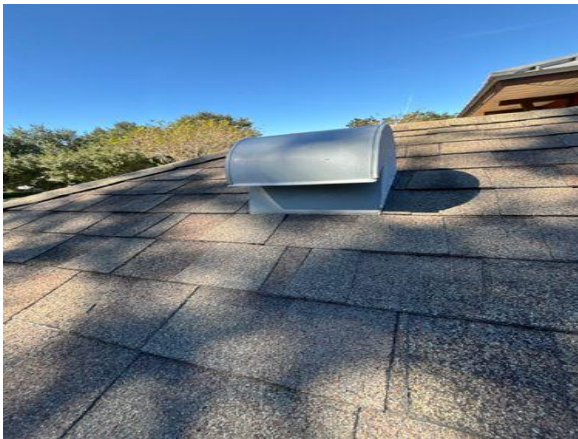
Example of goose neck penetration
