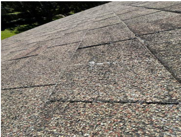
Fibers showing through shingles
