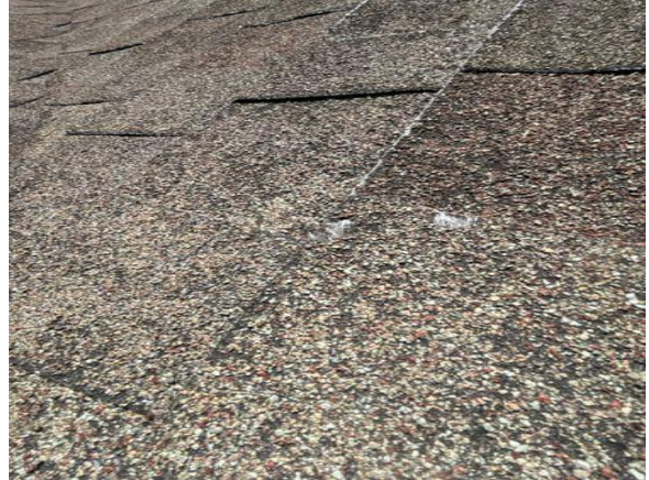
Fibers showing through shingles
