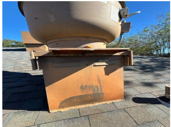
Missing grease pan
