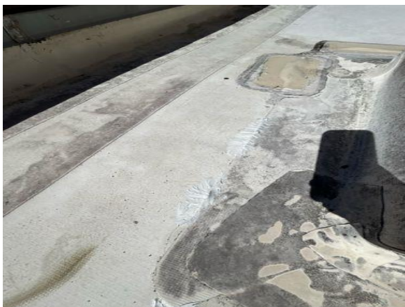
Loose flashing caulked
