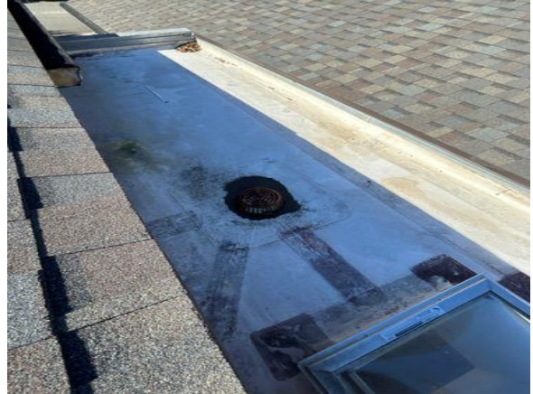
Example of drain penetration
