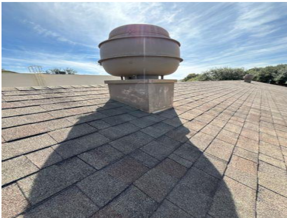
Example of vented penetration
