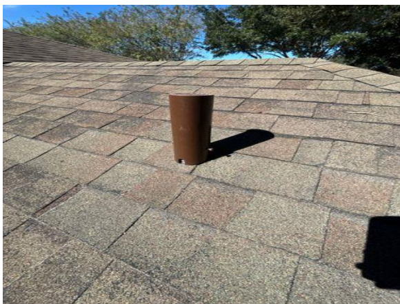
Example of pipe penetration
