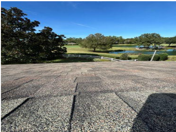
Example of general field and seams
