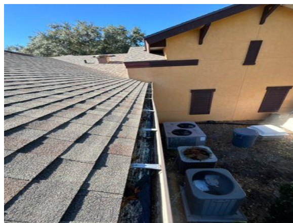
Debris removed and gutter unlogged
