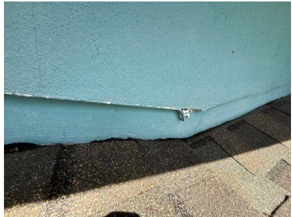
Deteriorating siding
