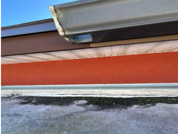
Missing downspout
