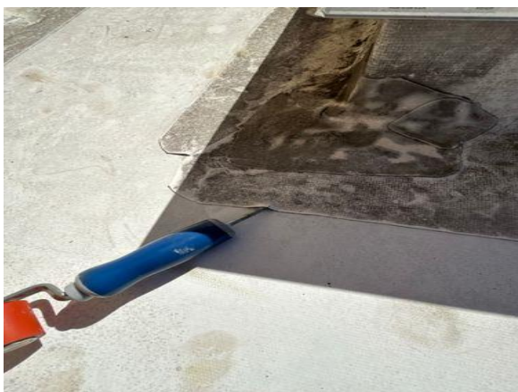
Loose flashing
