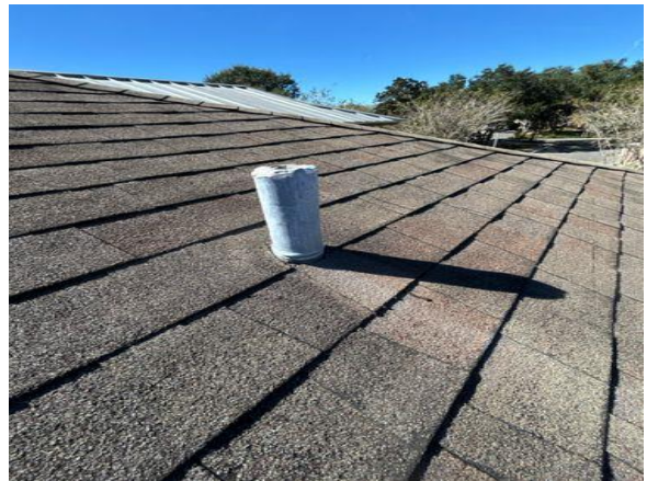
Example of pipe penetration
