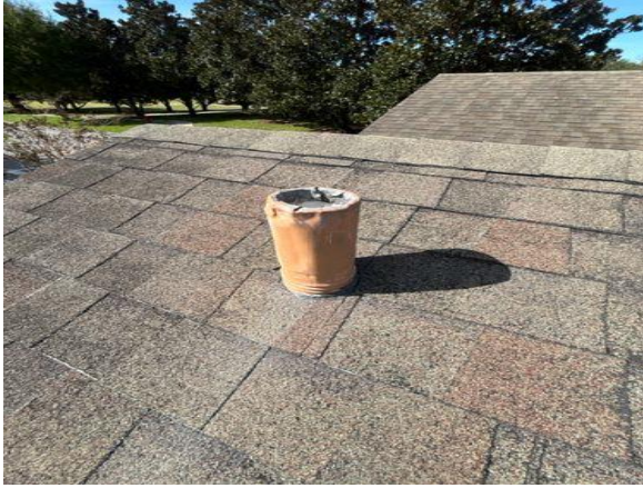
Example of pipe penetration
