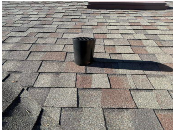
Example of pipe penetration
