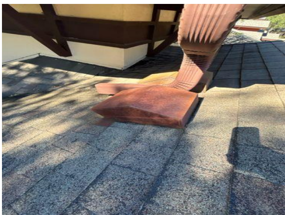
Example of goose neck penetration
