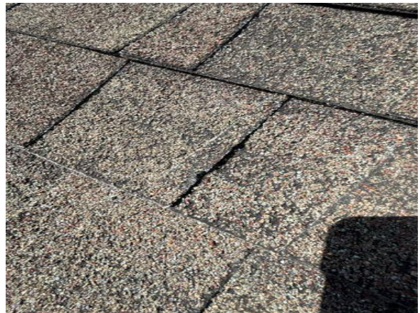
Worn down shingles
