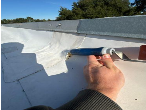
Loose flashing
