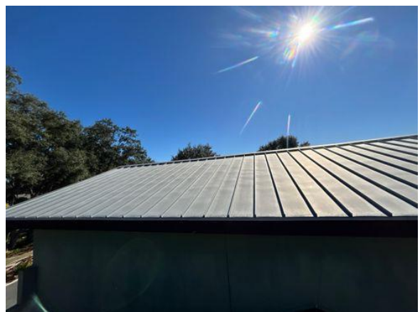
Example of metal general field and seams
