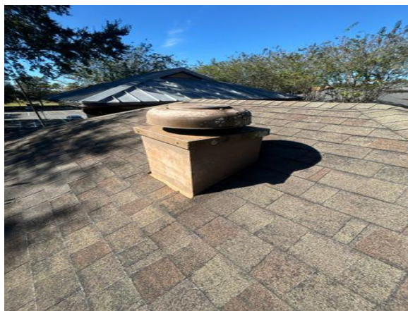
Example of big vented penetration
