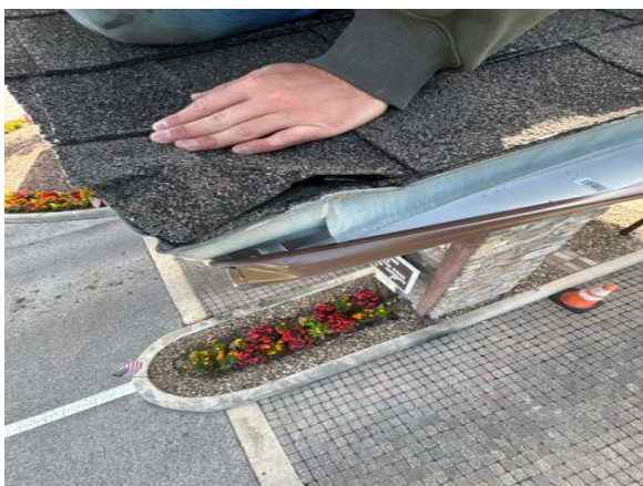
Crushed gutter
