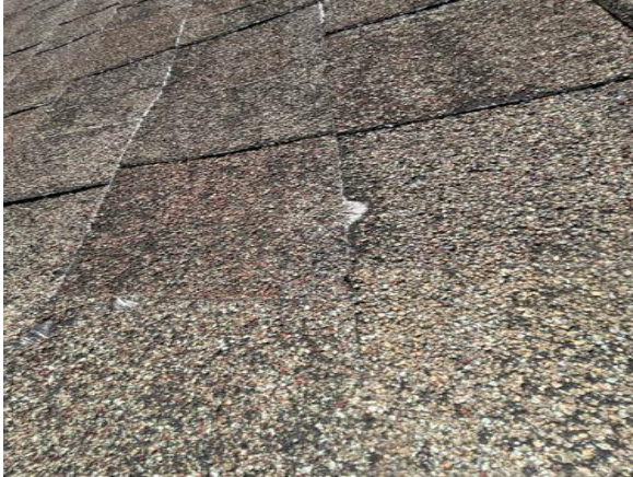
Fibers showing through shingles
