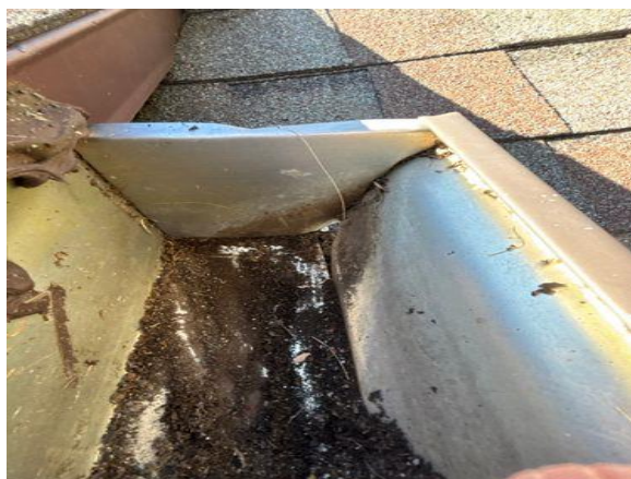
No downspout for gutter system. This gutter becomes a reservoir for water, running the risk of water backing up into building.
