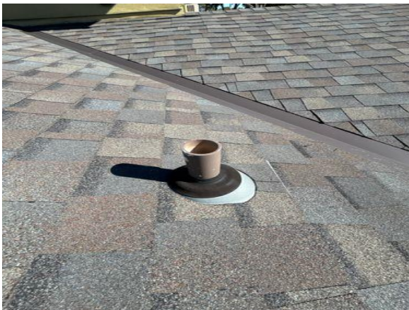
Example of pipe penetration
