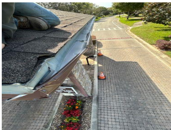
Crushed gutter
