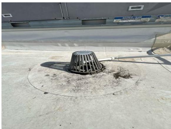
Example of drain penetration
