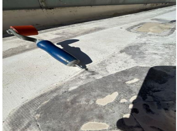
Loose flashing
