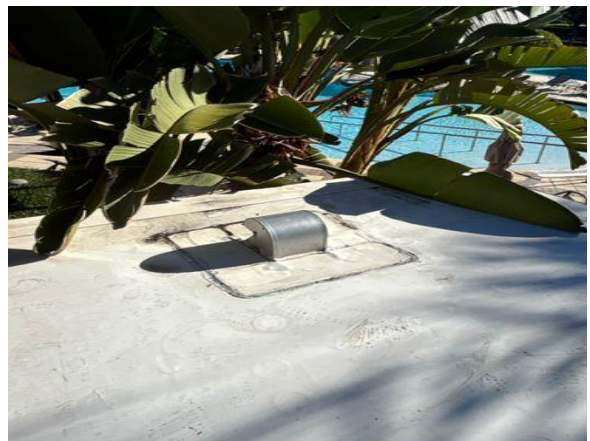
Example of goose neck penetration
