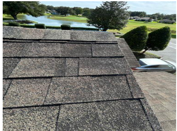
Shingles with granule loss
