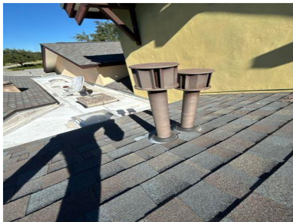
Large stack penetrations
