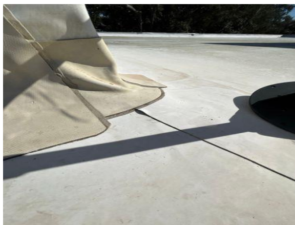
Loose flashing
