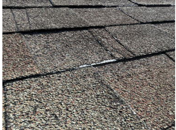
Closer look at worn down shingles
