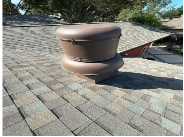
Example of vented penetration
