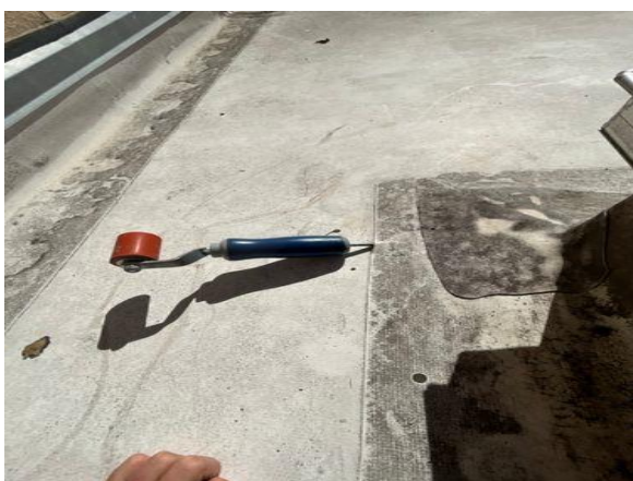
Loose flashing
