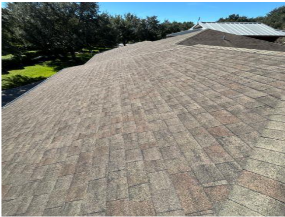
Example of general field and seams
