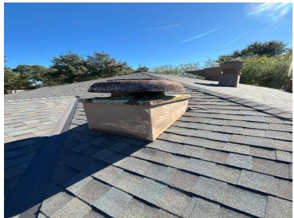
Example of large, vented penetration
