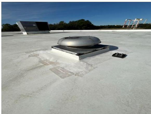
Example of vented penetration
