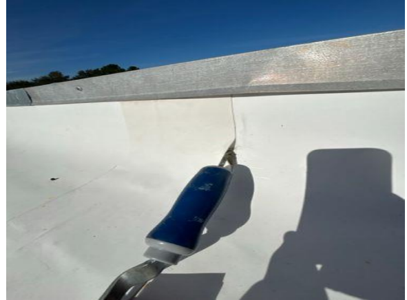
Loose flashing
