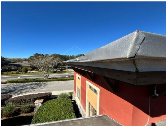
Example of metal edge perimeter
