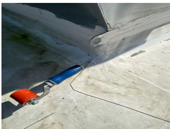
Loose flashing
