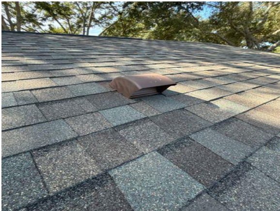
Example of goose neck penetration
