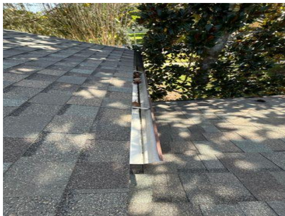
Missing gutter guards
