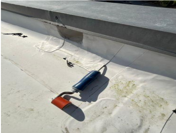
Loose flashing
