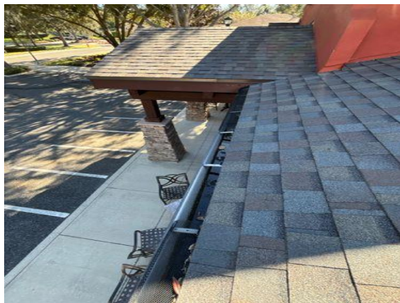
Missing gutter protector
