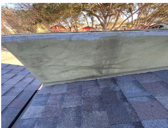
Cracking
