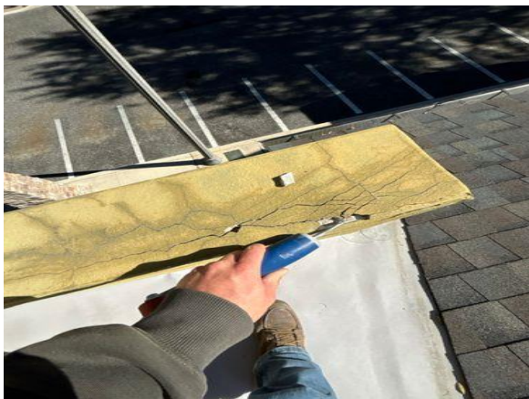
Cracking
