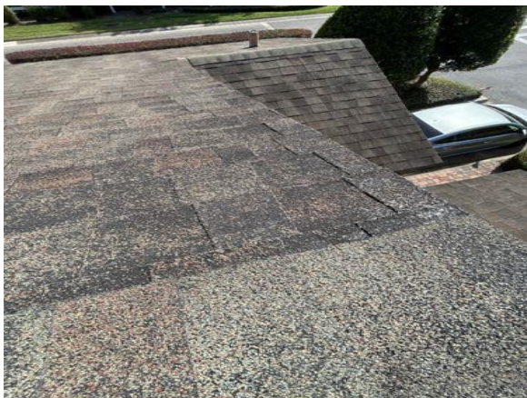
Shingles with granule loss
