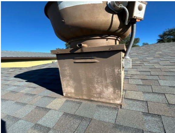
Missing grease pan
