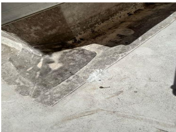
Loose flashing caulked
