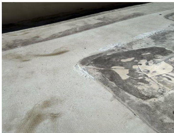
Loose flashing caulked
