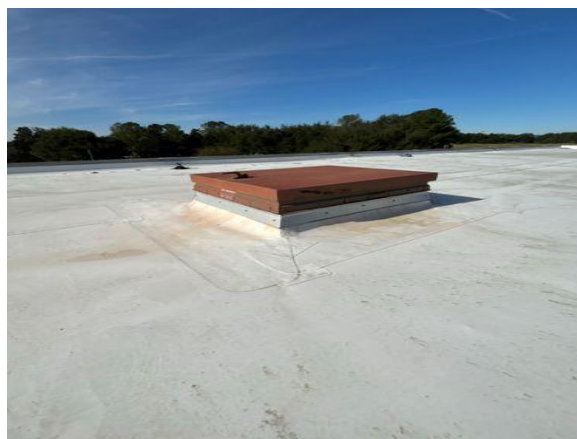
Example of roof hatch penetration
