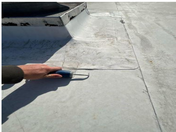
Loose flashing
