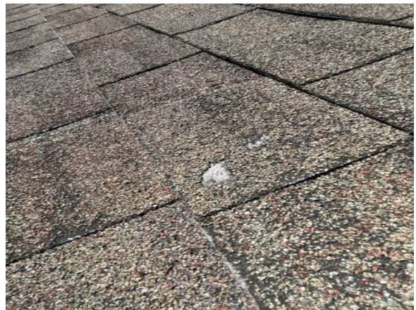
Fibers showing through shingles
