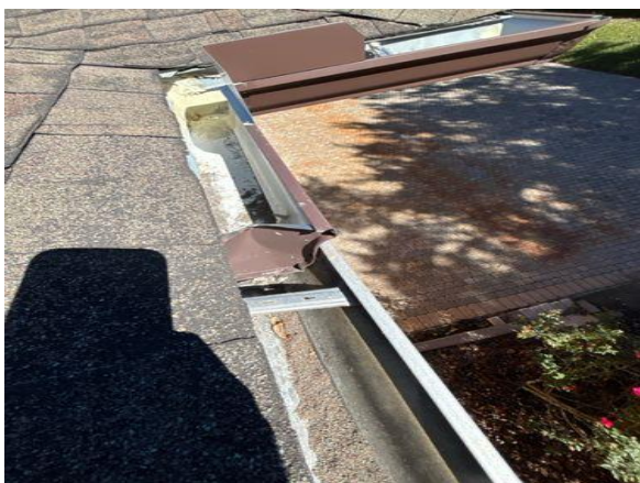
Not continuous gutter system
