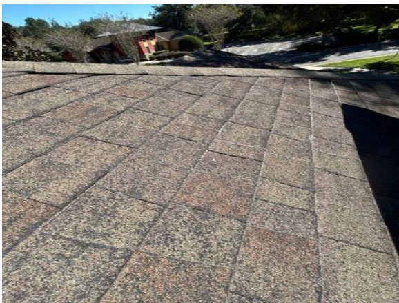
Weathered shingles
