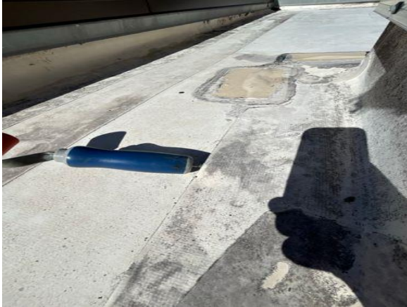
Loose flashing
