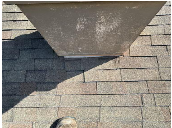
Slightly shifted shingles
