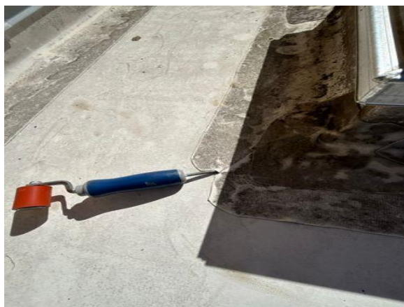
Loose flashing
