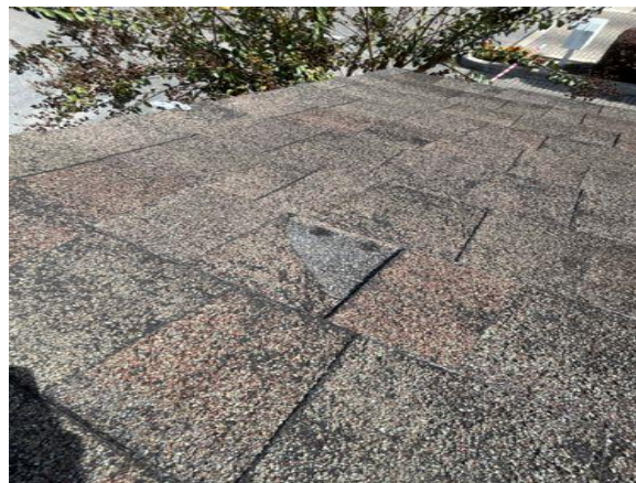
Damaged shingles
