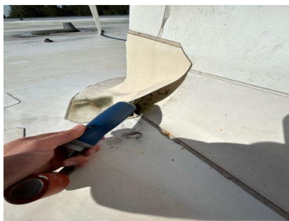
Loose flashing
