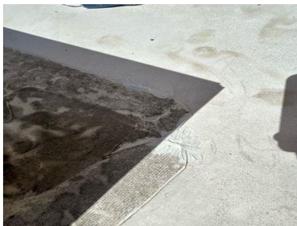
Loose flashing caulked
