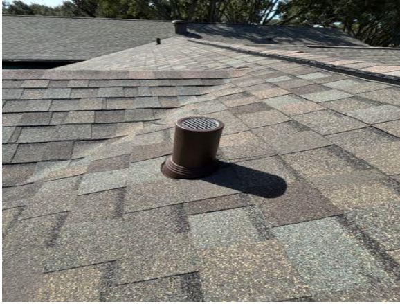
Example of pipe penetrations
